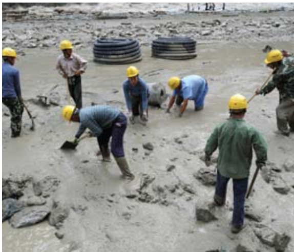
► GOVERNMENT REGULATION OF SILT runoff from construction sites isn't new, but stepped up enforcement practices in recent years are putting the risk on the radar screen of those who watch out for emerging environmental liability landmines.
